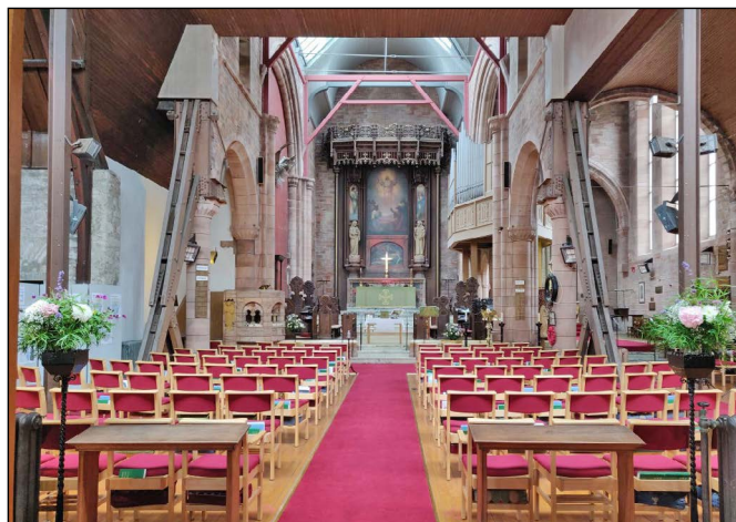
The Steel Buttresses Supporting the Tower (Picture from the Cathedral Website)
