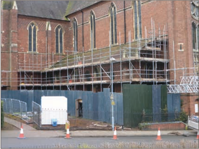
Scaffolding on the north side of the church
