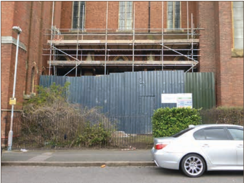
Scaffolding over the south aisle
